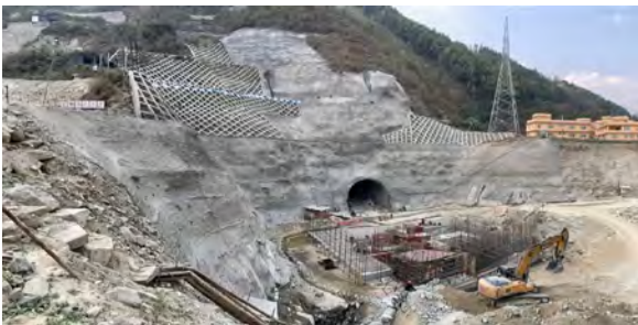
Construction work at Upper Trishuli 3B Hydropower (37 MW) Project
